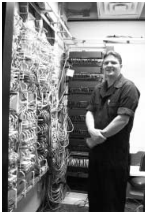
Network Analyst, Jason Dendy, in one of five Welch Hall wiring closets
